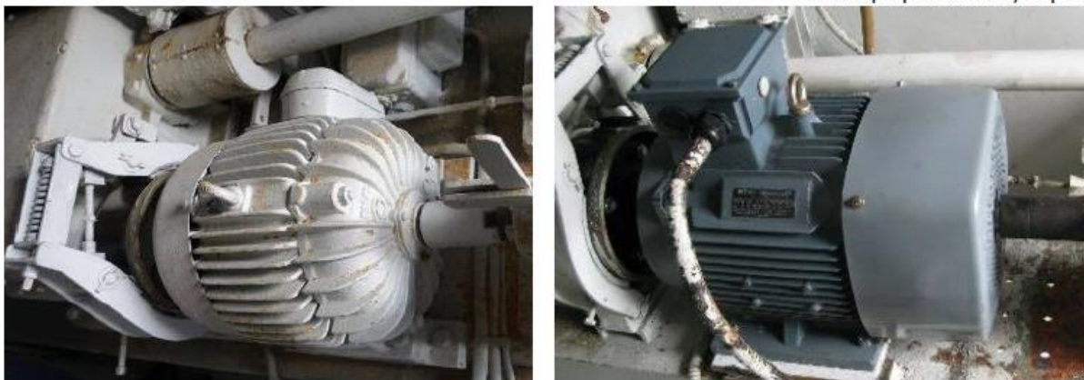
Figure 24: The outdated engine (left) was replaced by a new one (right)
