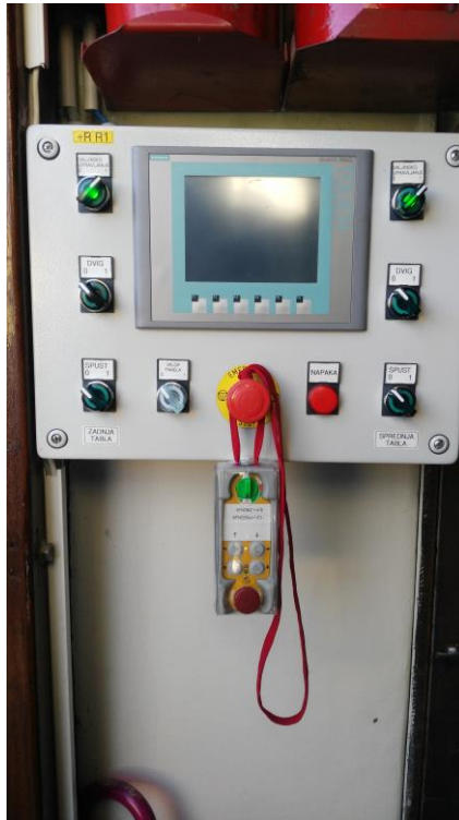
Figure 25: The touch screen displaying the position of the (right) barrier.
