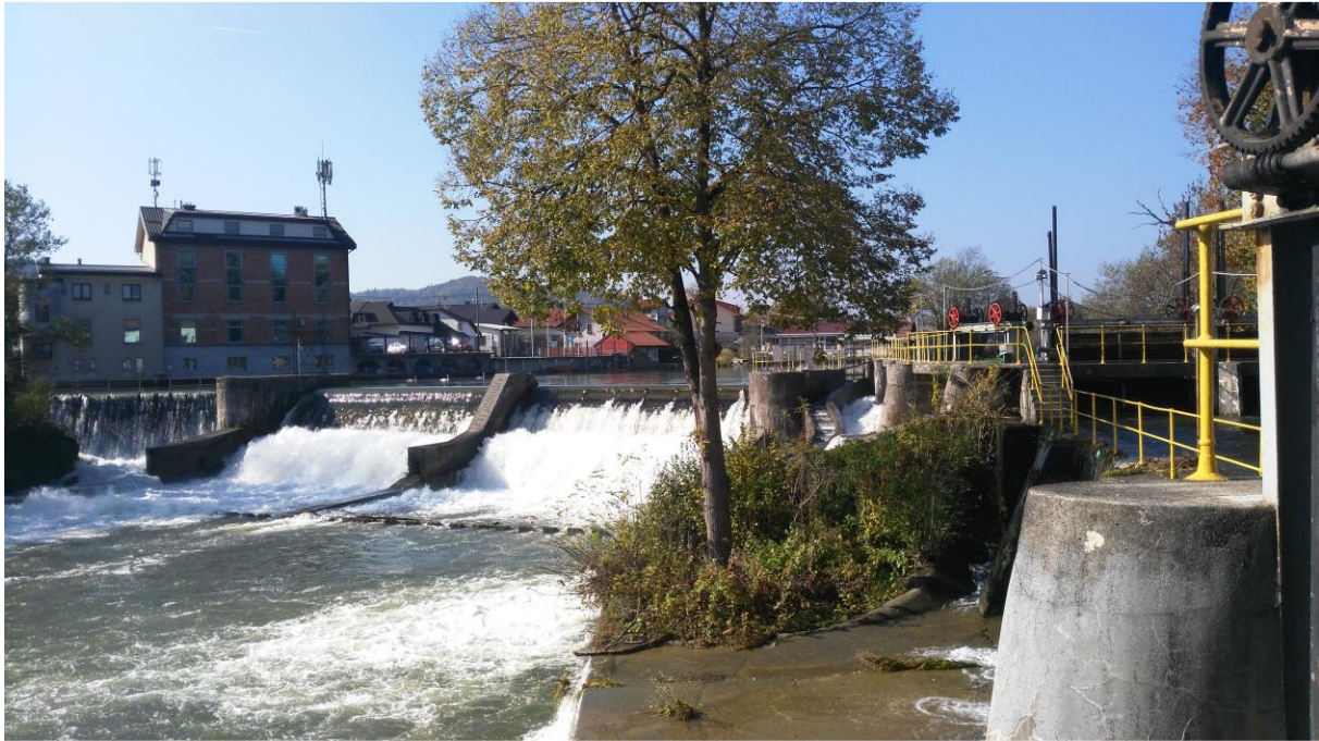
Figure 22: Weir at Fužine (left) and fish pass (right) after reconstruction works
