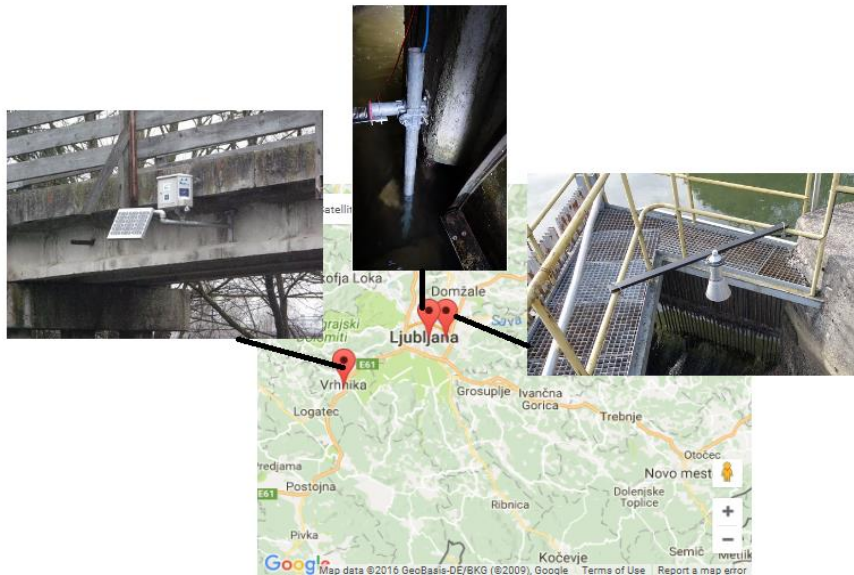
Figure 14: Locations of 3 online water stations and measuring equipment
