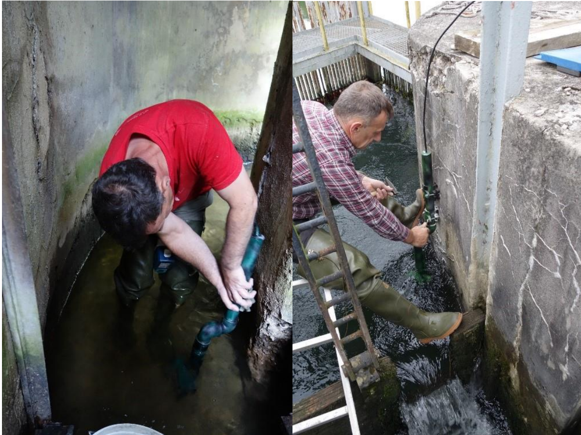
Figure 27: Installation of the fish monitoring camera in the fish pass at Ambrožev trg (left) and at the fish pass at Fužine (right).
