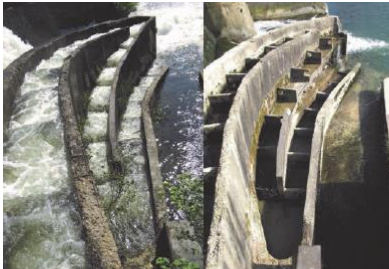
Figure 21: The fish pass at the Fužine weir prior to the restoration and its collapse (left) and after the collapse in autumn 2013 (right).
